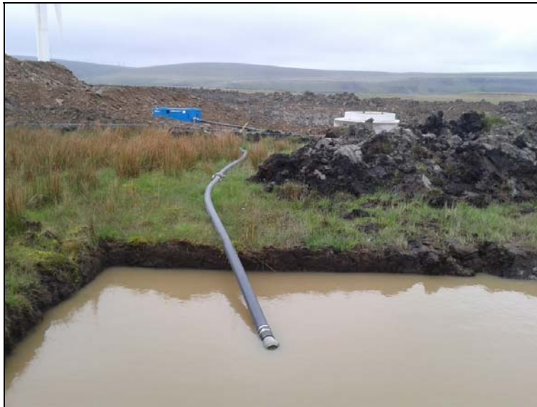
Plate 6: Typical 'Siltbuster' and settlement lagoon
