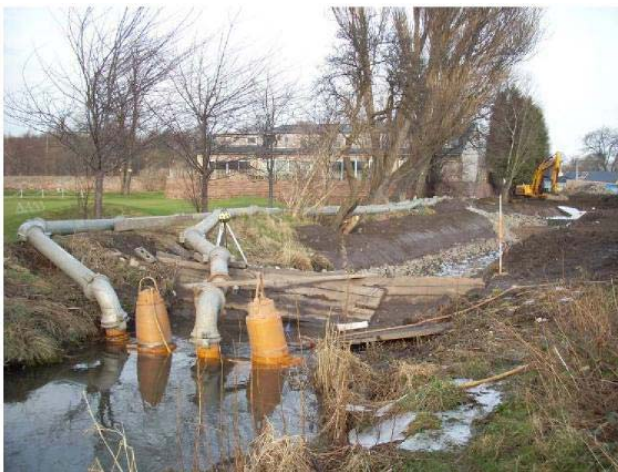
Plate 8: Full isolation – over pumping/siphon
